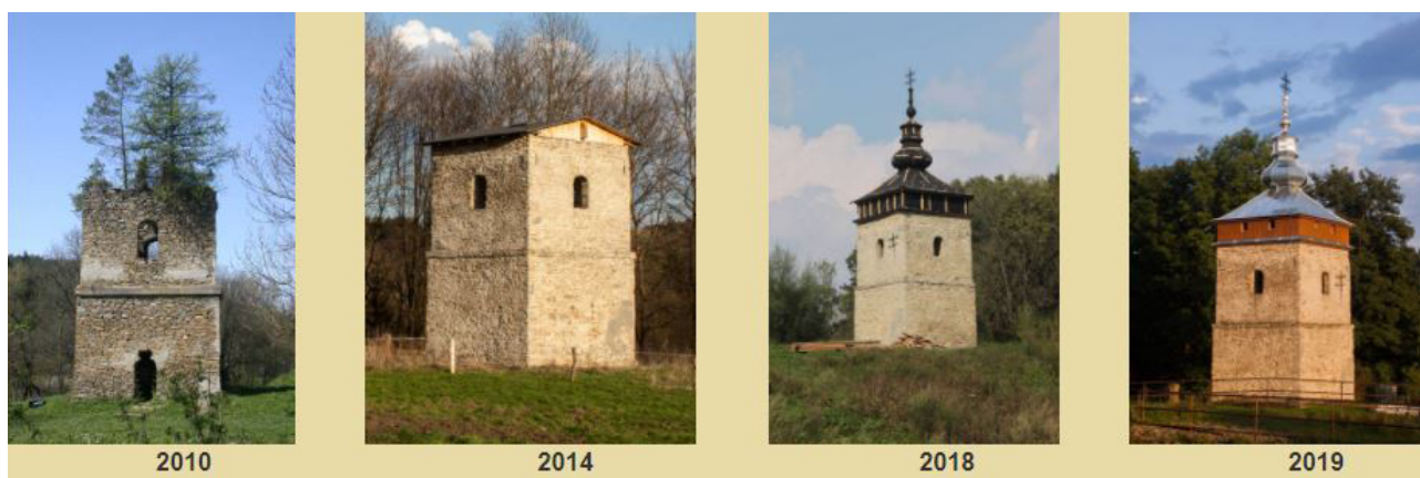
Fig. 23. Phases of the renovation of the bell tower in Polany Surowicze, http://polanysurowicze.waw.pl [accessed: 14/04/2022].
